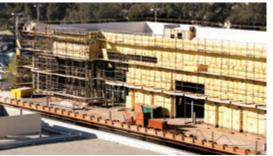
A southwest view of the Industrial Technologies Building. The yellow exterior on the facility serves as a moisture barrier, which allows interior work to continue during the rainy season.
